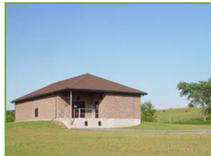
A community of 100 homes is serviced by this ROTORDISK® plant. It provides effluent treatment and advanced nitrate removal under one roof.
